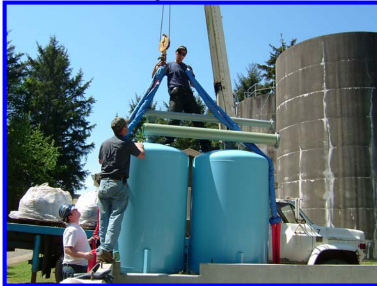
Crane unloading filters
