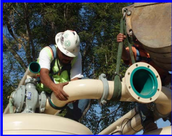
Connecting the influent manifold
