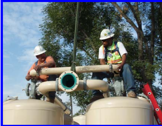
Connecting the backwash manifold
