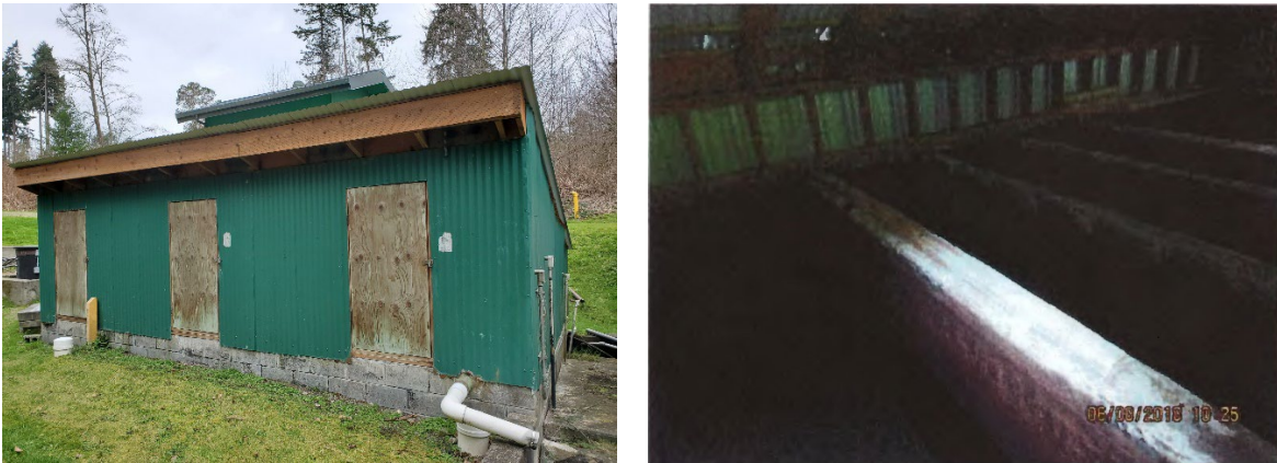
Figure 2.5 Baffled Chlorine Contact Tank
